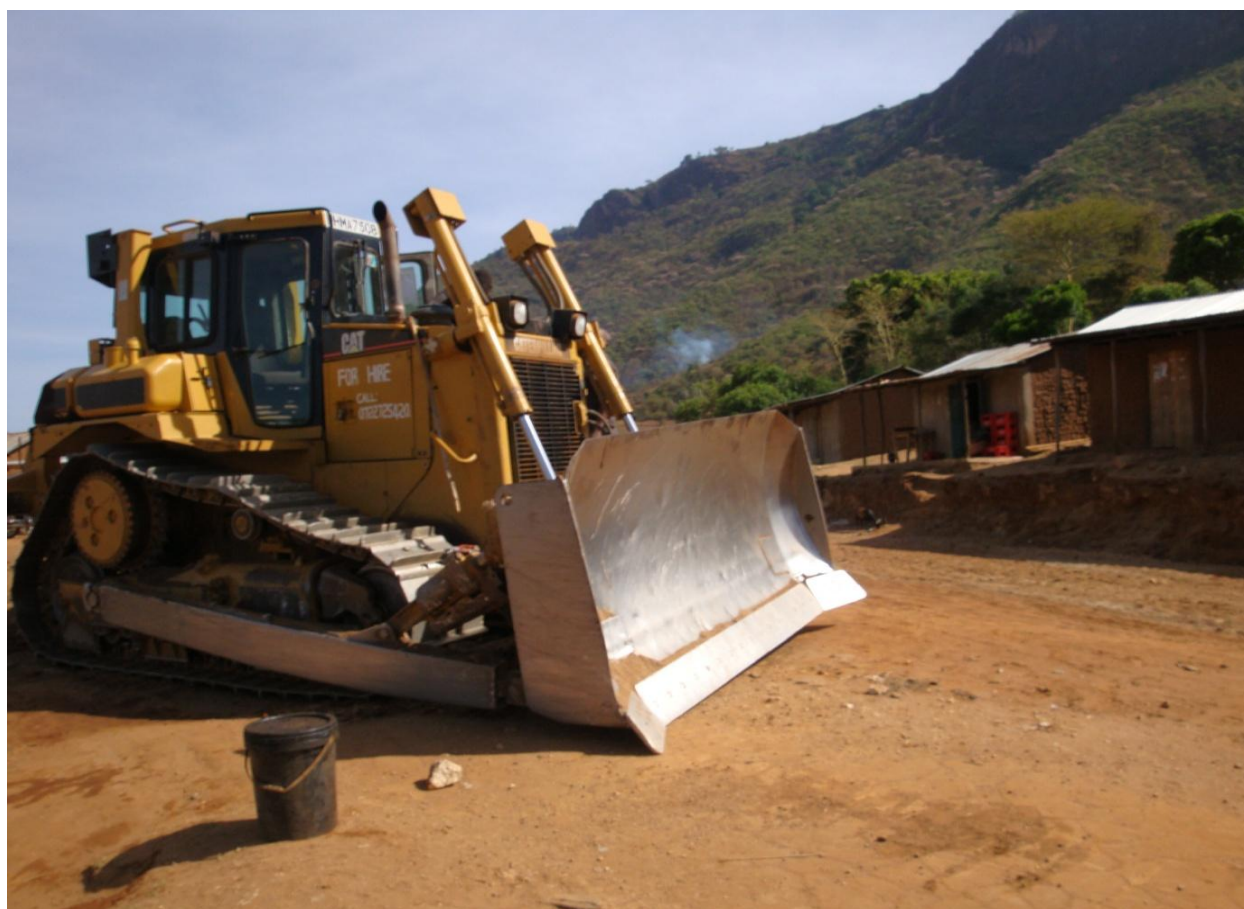
Figure 4.9: A Road to Kriich under Construction
