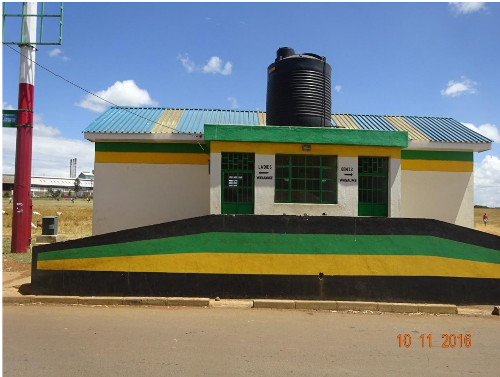
Figure 4.31 Ablution Block at Huruma
