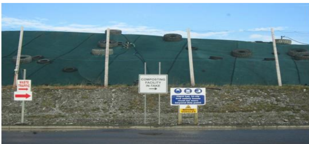
Figure 2.5: A well-managed sanitary landfill in the City of Dublin
