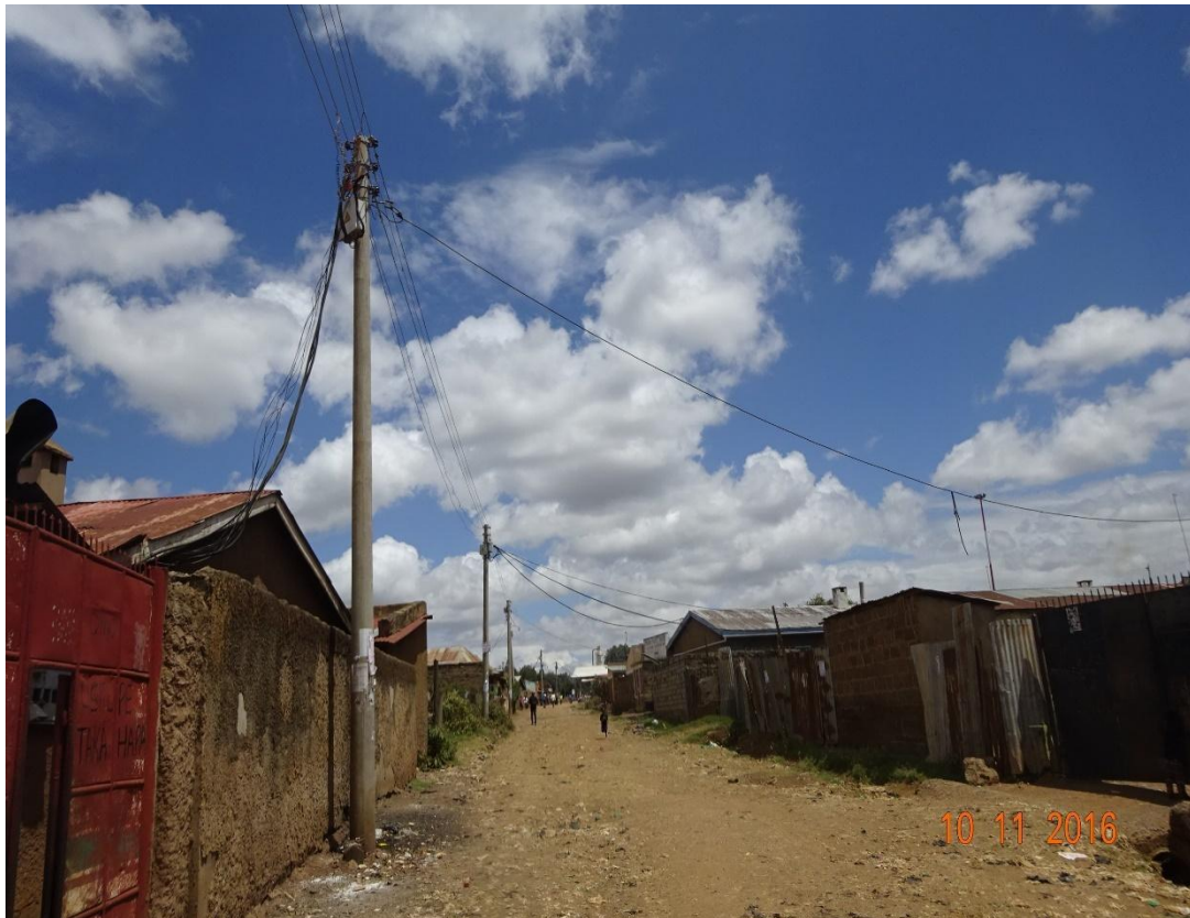
Figure 4.7: Electricity connection in some parts of Huruma
