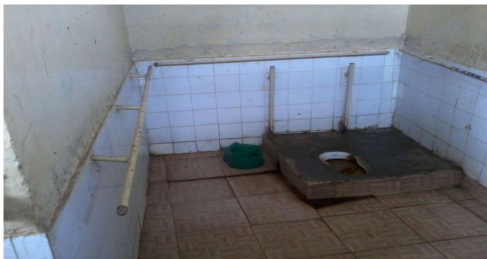
Figure 3: Presence of Adapted toilets with Holding Rails Used by Pupils with Physical Challenges
