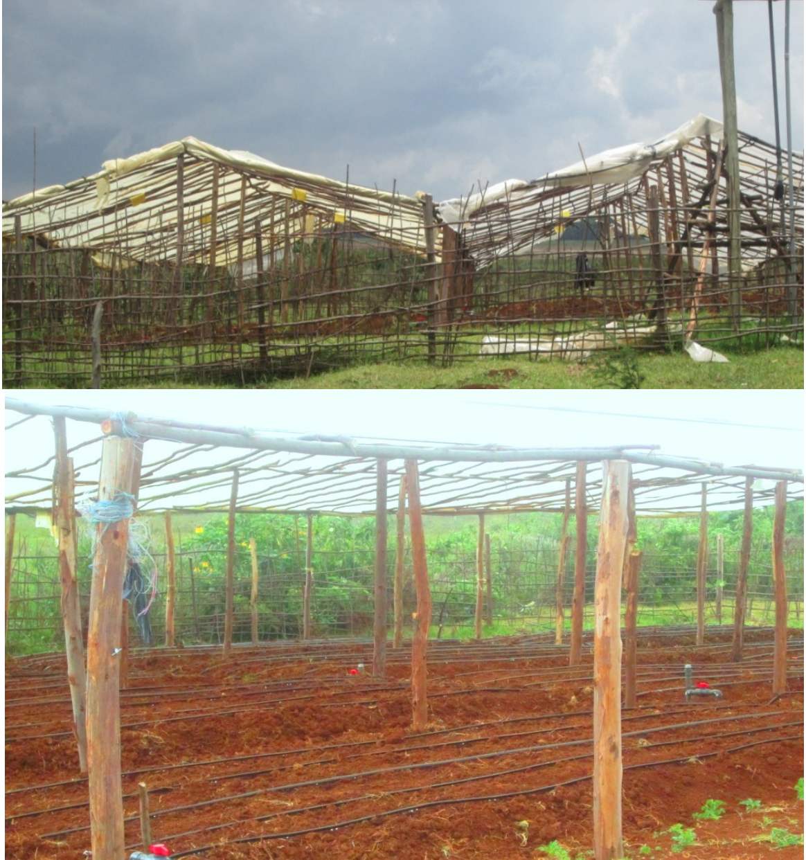
Plate 3.1: Rain shelter structure: (a) outside, (b) inside.
